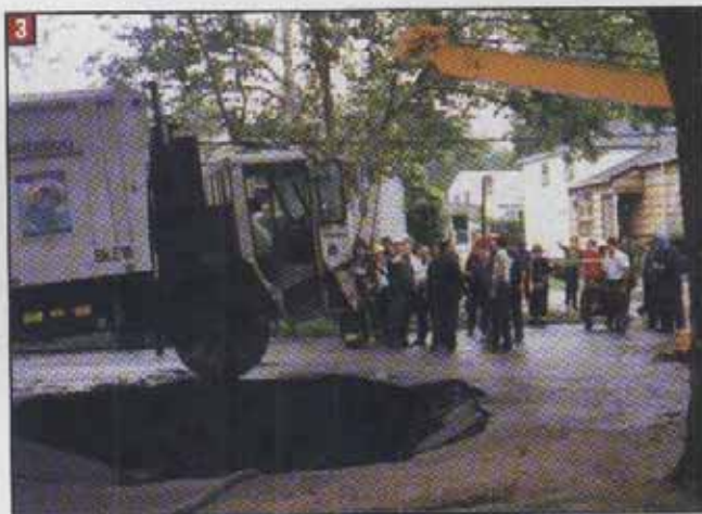
(1) The sanitation truck continued to sink into the hole as more and more of the pavement was undermined and collapsed. (Photos by author.) (2, 3) A large wrecker with a boom lifted the front of the truck while a smaller sanitation wrecker held the rear of the truck in place to prevent it from slipping into the hole. The boom operator then swung the cab onto stable ground.
