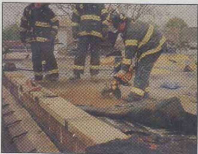
(Top left) EPDM roofing held in place by a metal fastener. (Right) Mod bit membrane roof being torched in place. (Bottom left) Firefighters cutting a mod bit membrane roofing on a Q-deck roof. First, they cut the membrane, then they must cut and pull up the fiberboard insulation. It is an arduous, labor-intensive task. The fiberboard smoldered and spread underneath the membrane. Cutting and pulling over a large area was required to ensure extinguishment.
