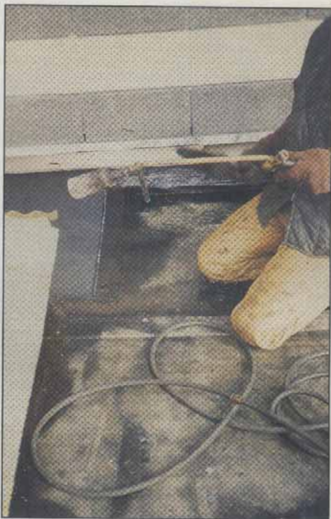
(Top left) EPDM roofing held in place by a metal fastener. (Right) Mod bit membrane roof being torched in place. (Bottom left) Firefighters cutting a mod bit membrane roofing on a Q-deck roof. First, they cut the membrane, then they must cut and pull up the fiberboard insulation. It is an arduous, labor-intensive task. The fiberboard smoldered and spread underneath the membrane. Cutting and pulling over a large area was required to ensure extinguishment.
