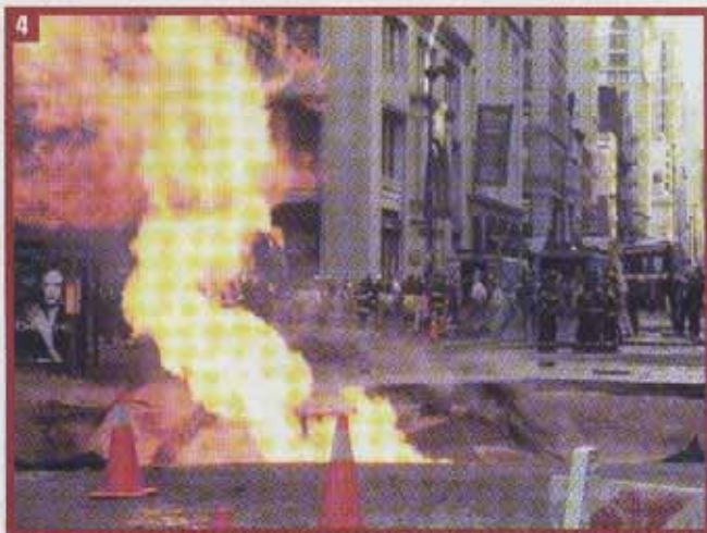
(4) A water main break severely undermined the street. The undermined gas main broke and the escaping gas ignited.
