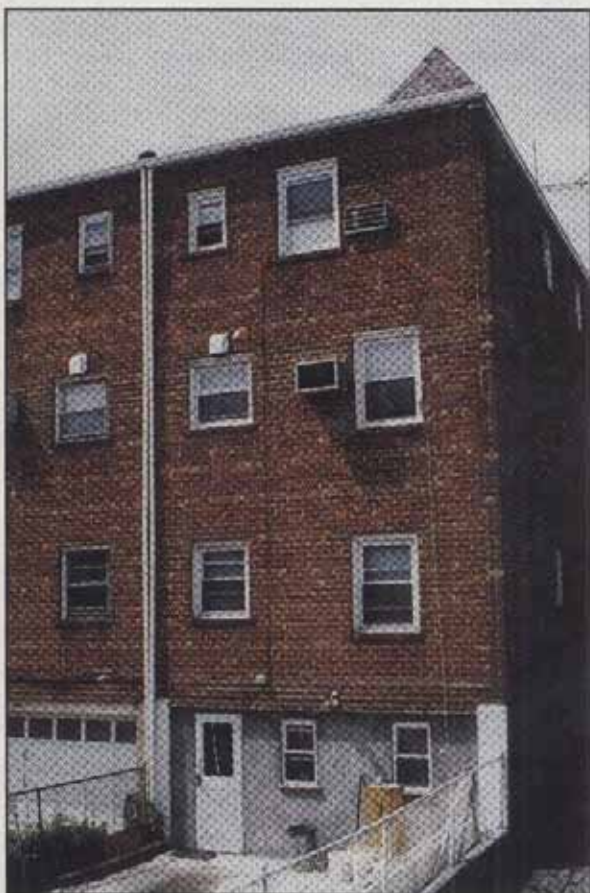
However, when viewed from the rear, with the grade-level as the first floor, this is a four-story building.
