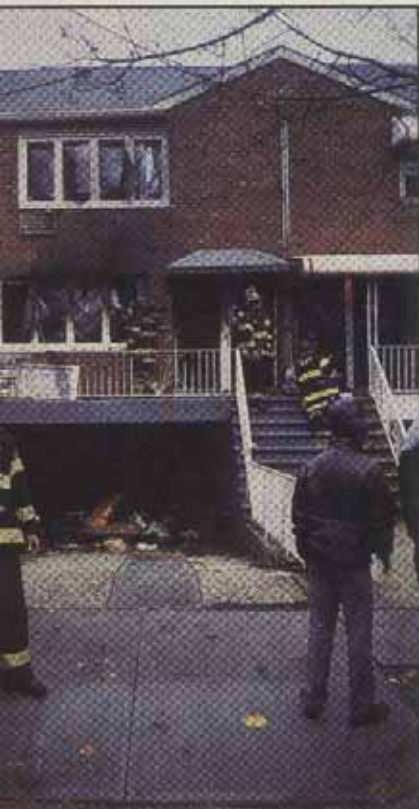
At a fire in this building, there was confusion as a result of the split-level layout of the second and third floors. Note: The garage is on the basement level and is designated as the first floor.
