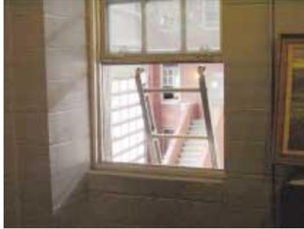
*(2) An improperly placed ladder blocks exiting from the window (interior view). Even if the upper sash and mullion were removed, it would still block egress.*
